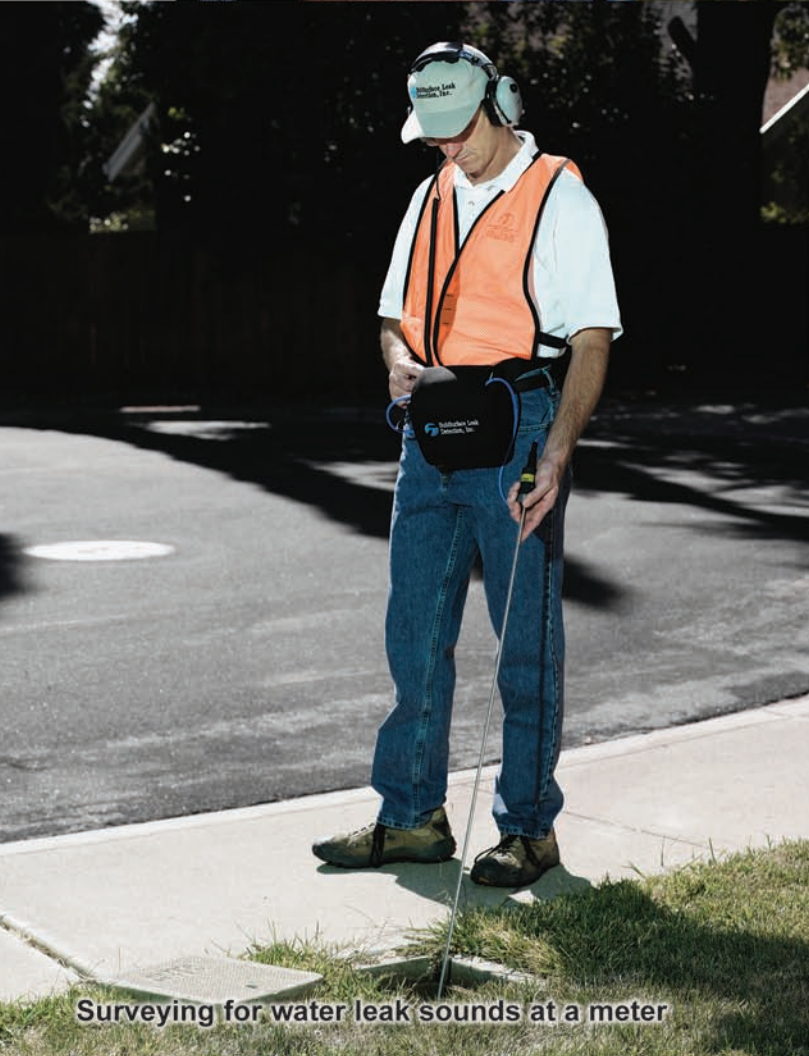
Displaying leak loudness at a water meter
